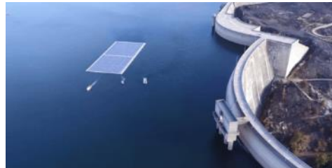
EDP S.A. , photo by Pixbee – Floating solar on Alto Rabagão hydro dam in Portugal
