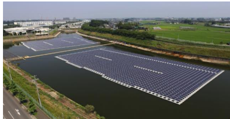
NIKKEI , 2013, 1.2 MWp floating PV system at the Okegawa in Japan
